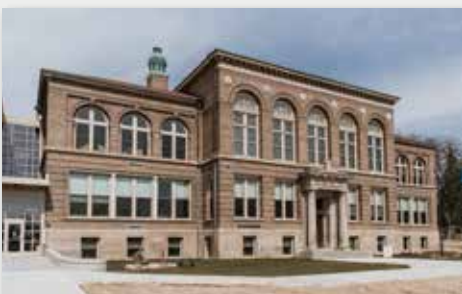
Wgechda Renovation at Wegma Campus Formerly Albrecht Hall
