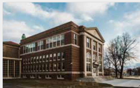
Wgechda Renovation at Wegma Campus Formerly Rickner Library
