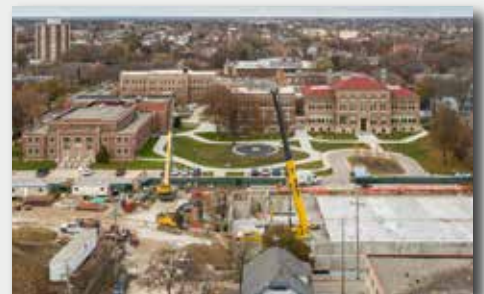
Wgema Parking Structure
