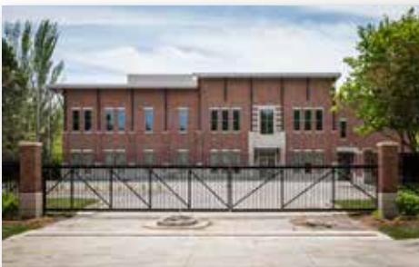
Data Holdings – Generator Expansion
