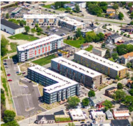
Stitchweld Apartments $36 million new construction of a four-building, 241 unit apartment community totaling 320,000 SF.
