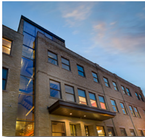
NO Studios, Phase II $3 million interior build-out of a 40,000 SF office building in Milwaukee's newly redeveloped Historic Pabst Brewery complex.
