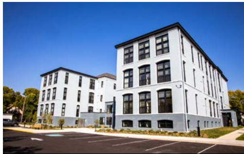
37TH STREET APARTMENTS
