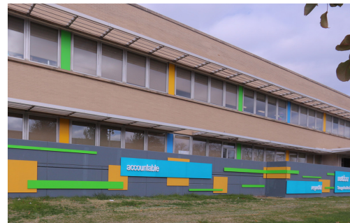
NEXT DOOR FOUNDATION
