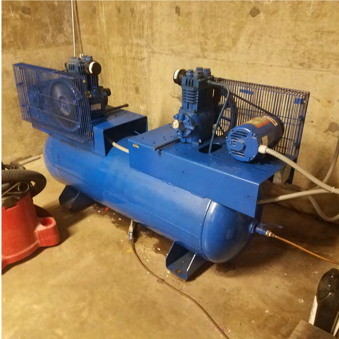
Compressor to control pneumatic thermostats
