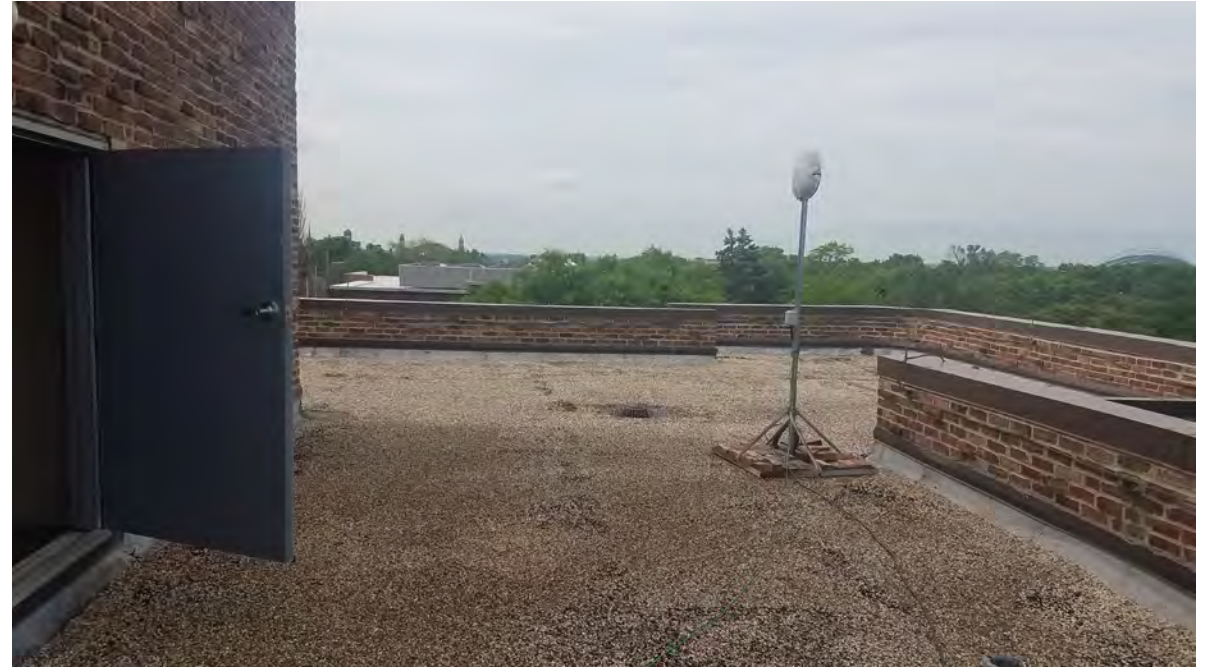
Membrane and ballast roof
