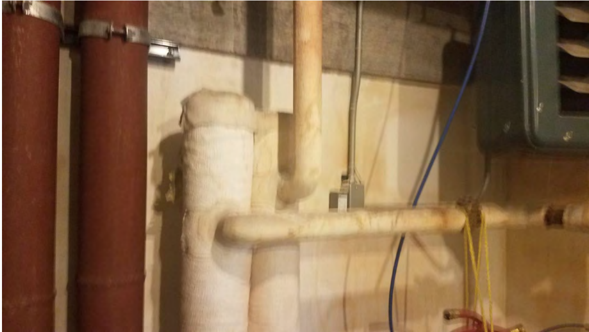
Potential asbestos-containing pipe wrap
