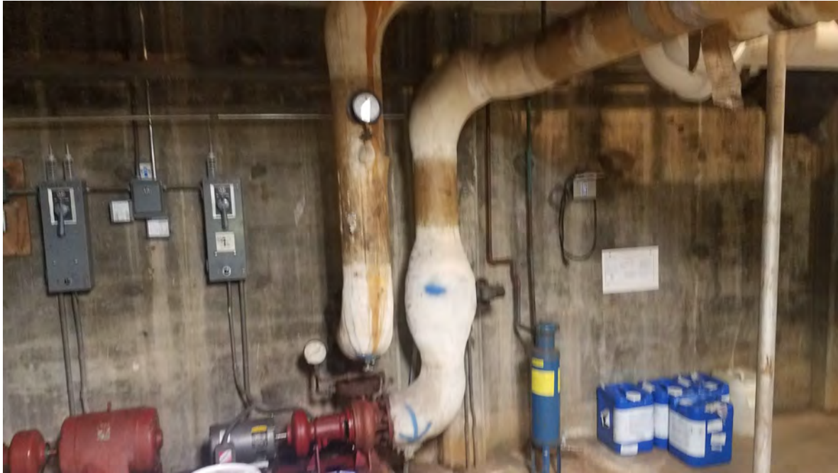
Fire pump piping and potential ACM pipe wrap
