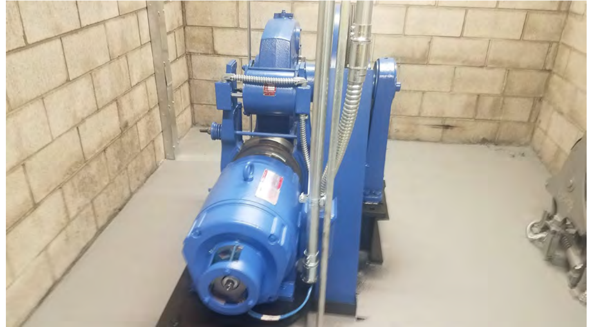
New elevator motor
