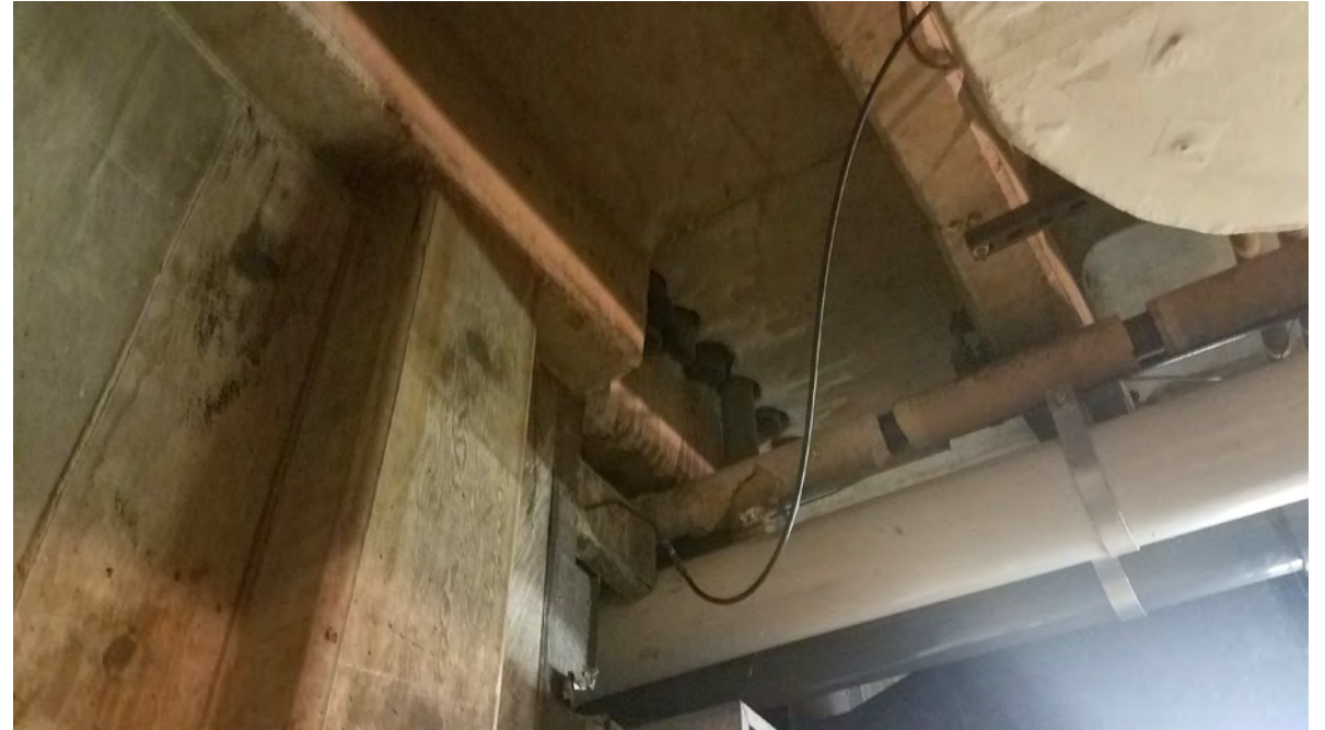
Piping through ceiling, possibly former fuel oil UST piping
