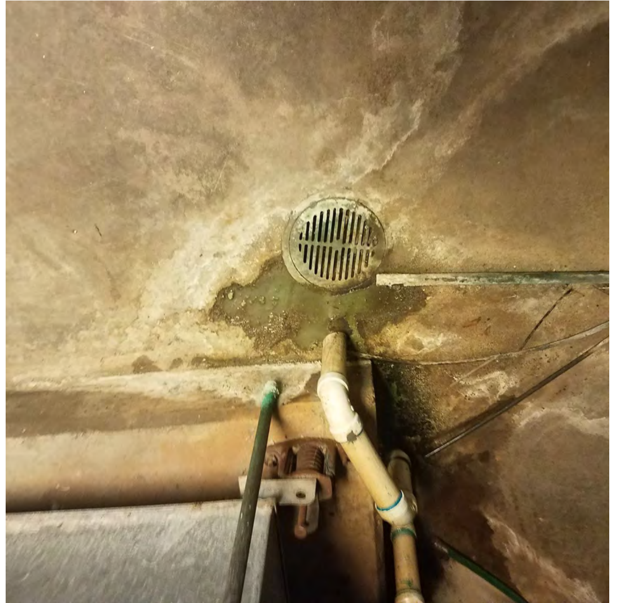
Boiler condensate drain
