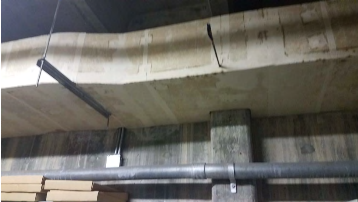
Basement duct work and potential ACM wrap
