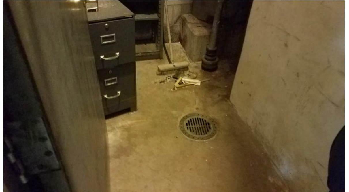
Basement floor drain
