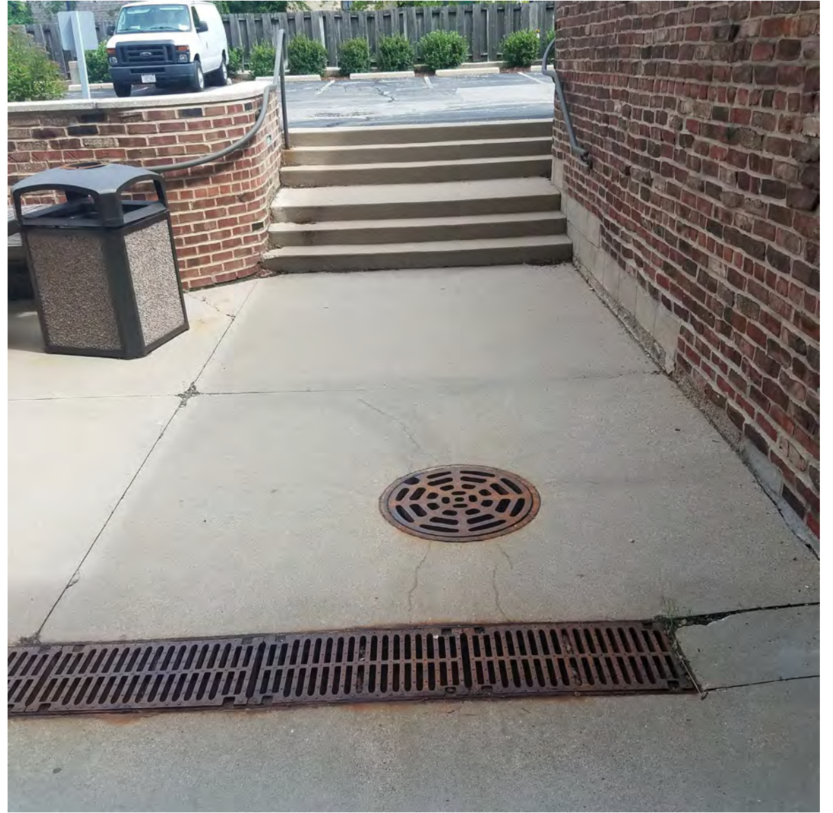
Catch basins at rear building entry
